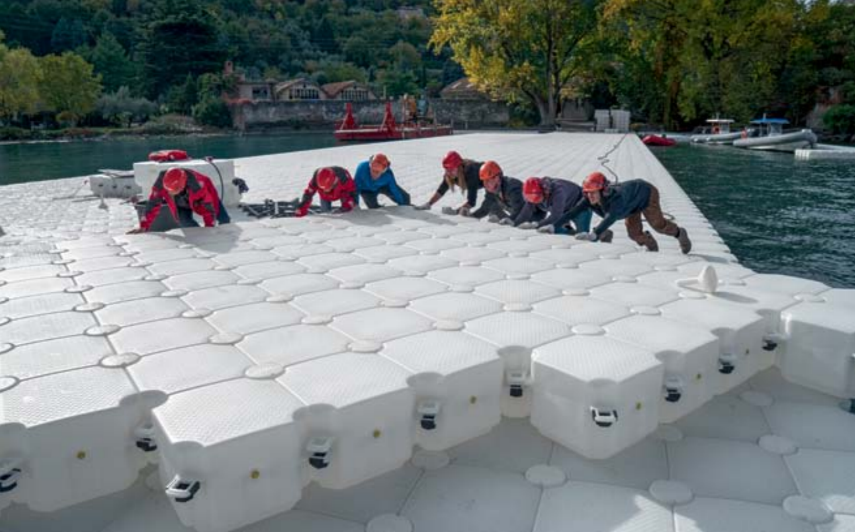
Above: A test of the angle attachments at Montecolino in November 2015.
